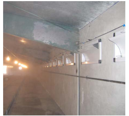
Nozzles above windows for cooling and humidification
